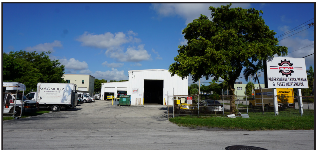
Professional Fleet Maintenance of Fort Lauderdale, Florida, has been an installer of JASPER remanufactured products for the past 15 years.
